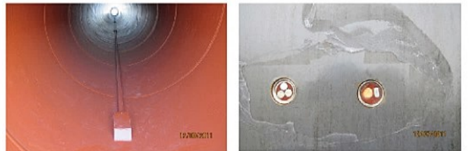
腐蚀监测探头安装与防护
